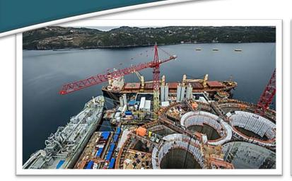
Iron ore bulk carrier (top) and fly ash bulk carrier (left) moored at the flotilla for installation of solid ballast in the Gravity Based Structure.
